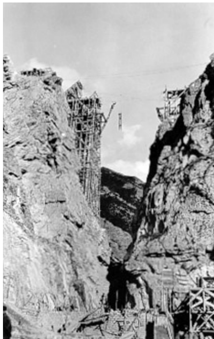
Photo 15: Operation that is to connect the two columns and construction of the curved slab are started.
