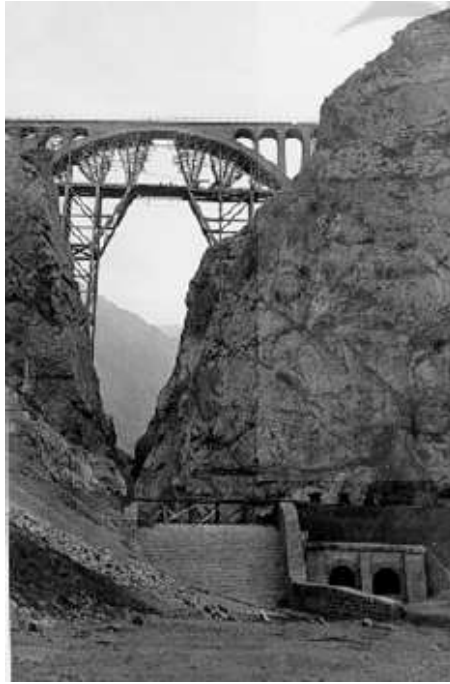
Photo 32: Completion of the underground tunnel
