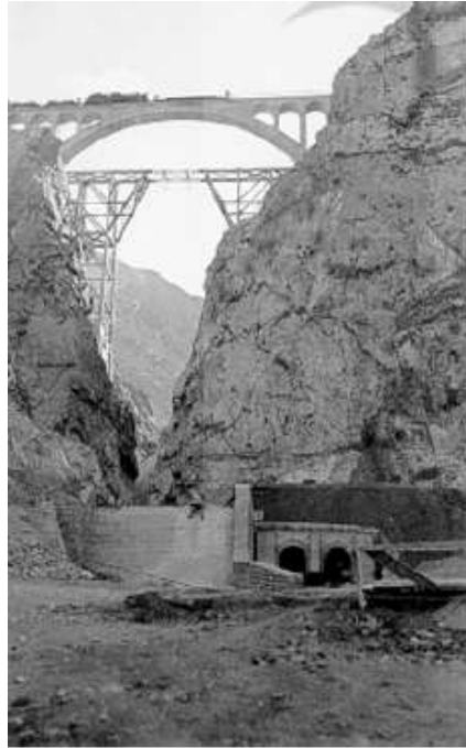
Photo 44: A view of the bridge, underground tunnel and water channel
