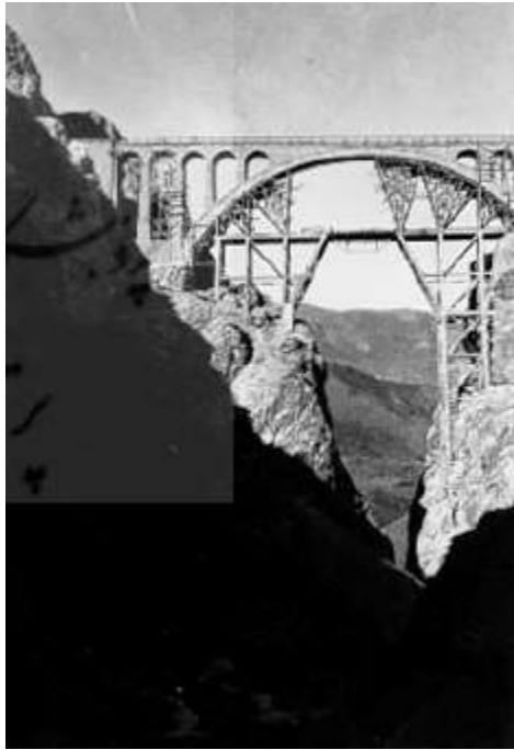
Photo 34: Construction of the brick bridge
