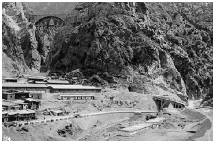
Photo 29: A view of Veresk Bridge and the upper pass railway bridge of Firoozkooh road.
