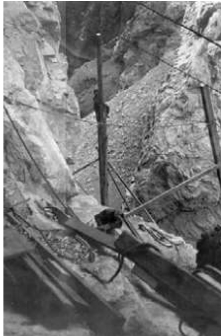
Photo 2: Transferring of materials and tools using two connected cables
