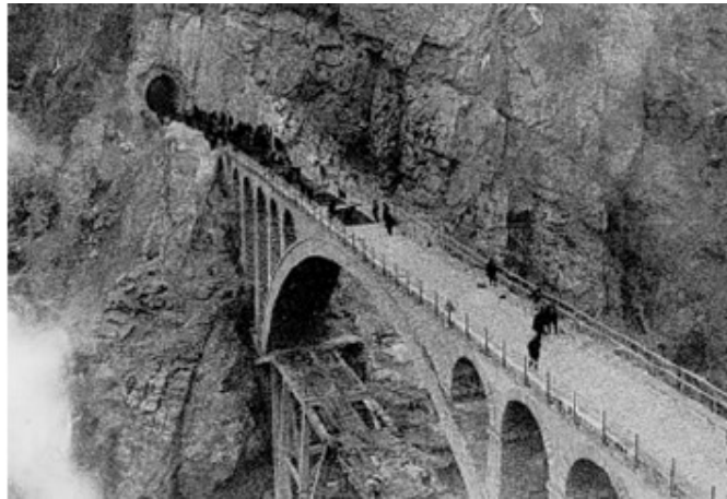
Photo 39: Preparation of the bridge to install ties
