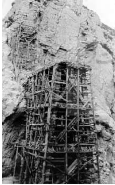
Photo 8: Another view of the stand construction
