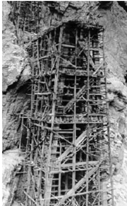
Photo 9: Another view of the stand construction
