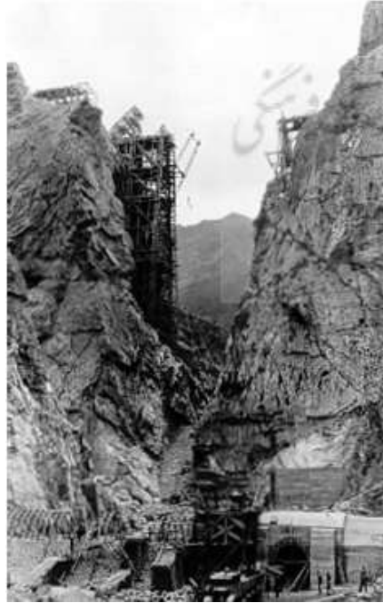
Photo 16: The concrete forming for the ceiling of underground tunnel is under construction.
