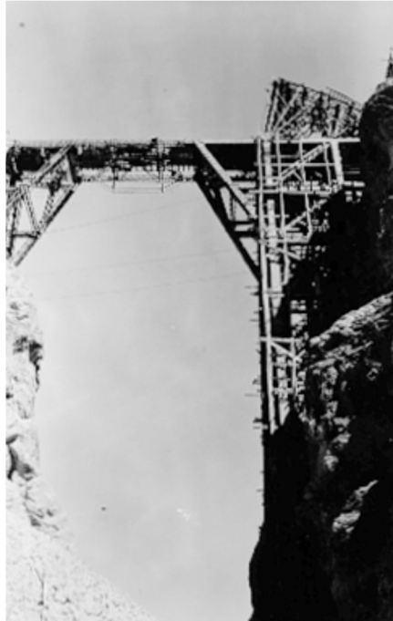
Photo 20: Two stands of scaffolds are connected to each other.
