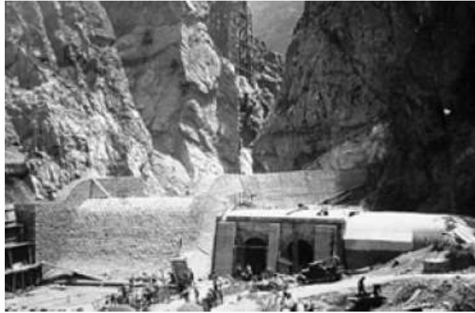
Photo 30: Last stages of the underground tunnel construction and water channel
