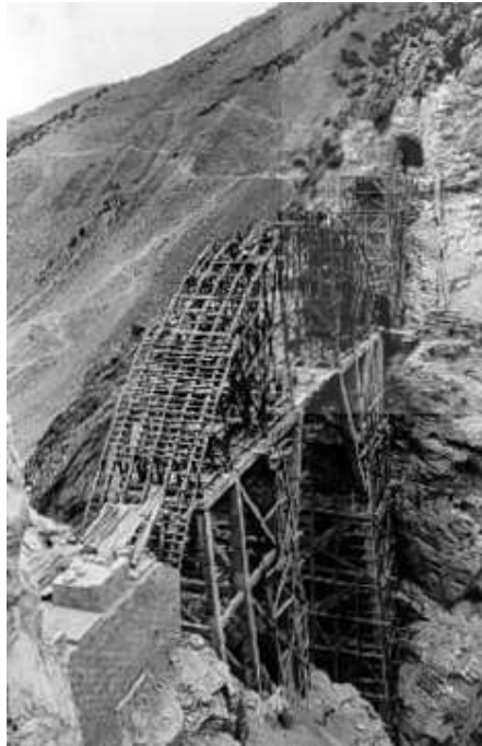
Photo 23: Two parts of curved slab are connecting to each other.
