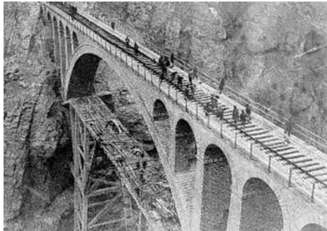
Photo 40: Installing ties and rails
