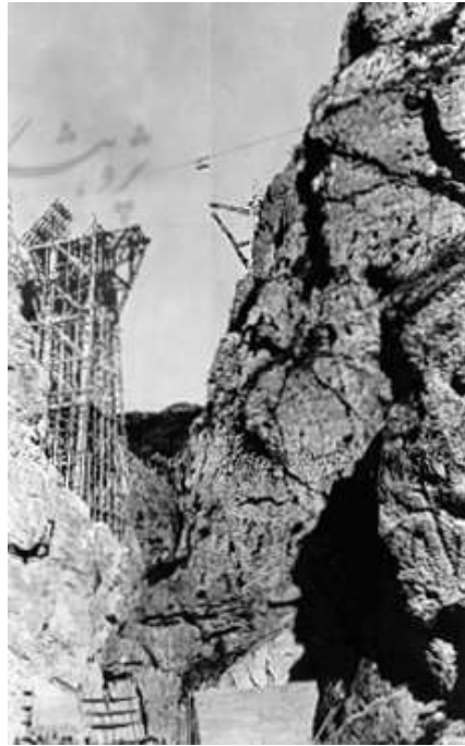
Photo 18: Transferring of materials and pre-cast elements using the cable.
