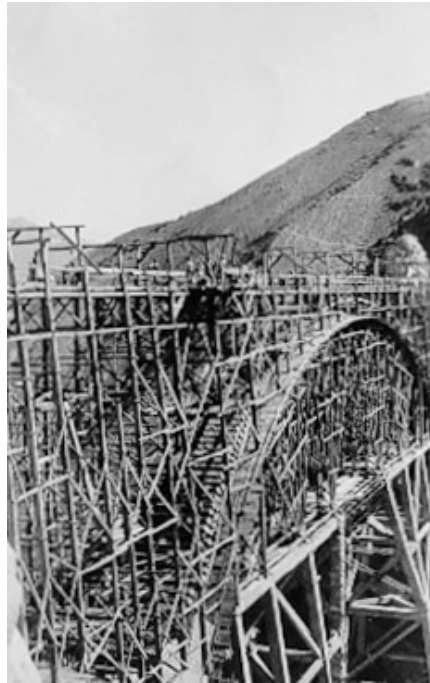
Photo 27: A view of the formed bridge.
