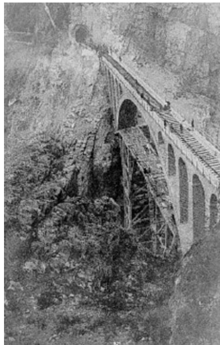
Photo 41: Installing ties and rails
