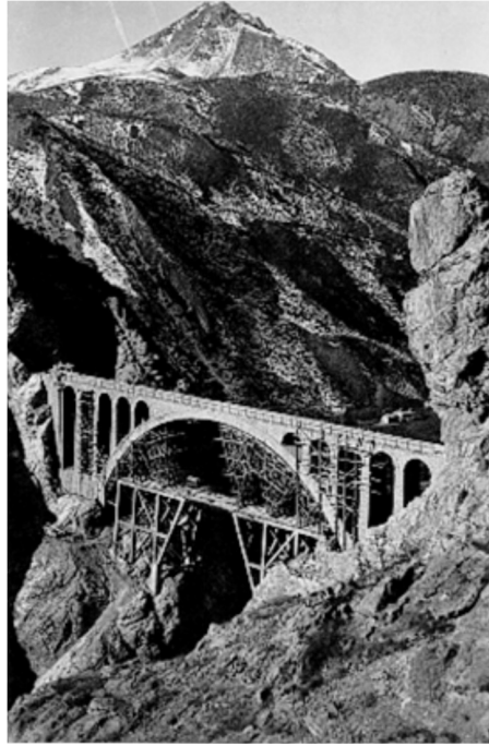
Photo 36: A view of the bridge and Damavand peak
