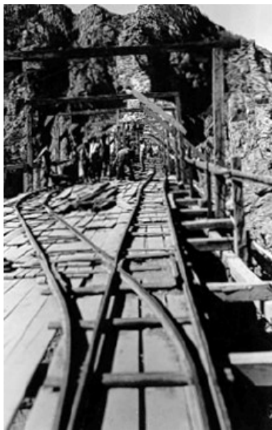
Photo 35: Temporary railing to facilitate the ongoing traffic on the bridge
