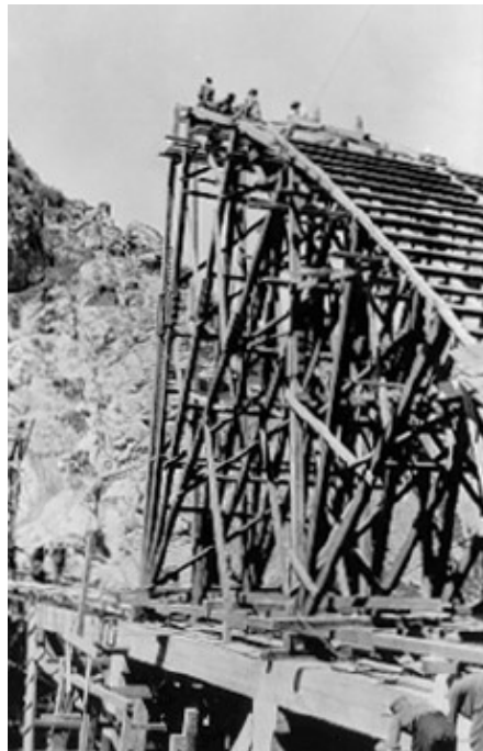
Photo 21: Workers are completing the forming of curved slab.
