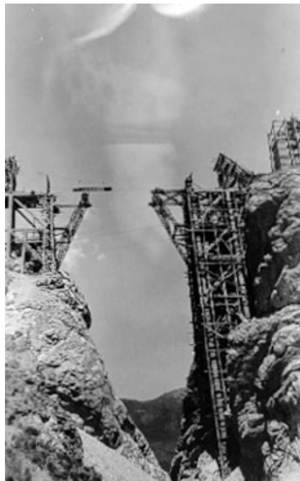
Photo 17: Transferring of materials and pre-cast elements using the cable.
