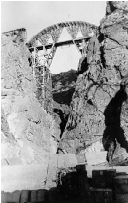
Photo 25: The completion of curved slab forming
