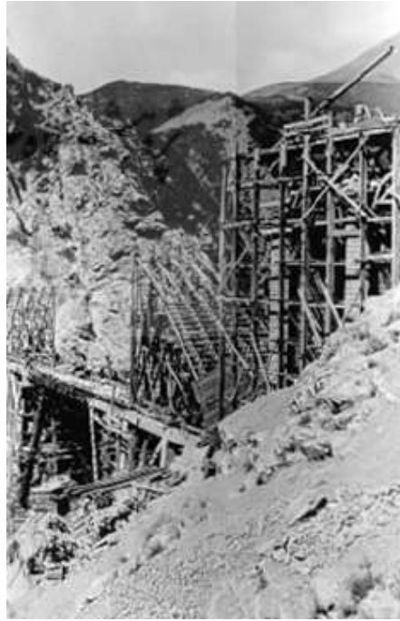
Photo 22: Another view of curved slab casting.
