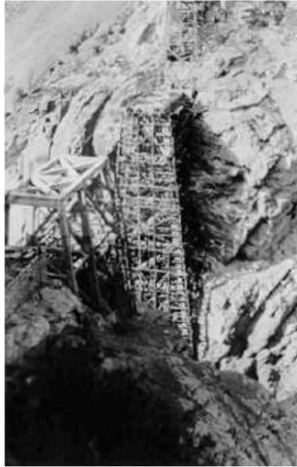
Photo 14: The taller concrete structure is under construction.
